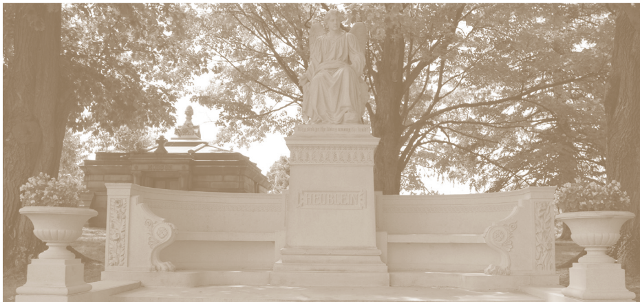
Monument Conservation Collaborative cleaned the Heublein Monument. They removed extensive organic growth, returning the exedra to its original glory.
