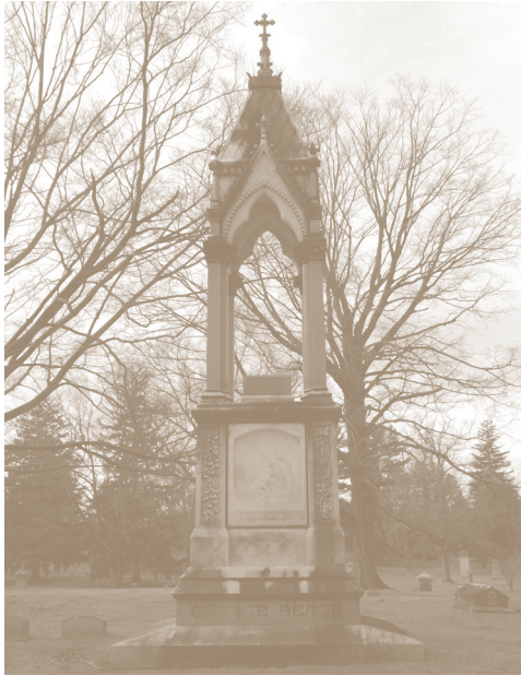
The Beach Monument in Section 2 is in need of restoration. A multi-year project to clean and stabilize the historic monument will address critical preservation concerns. Monument Fund donations will support this important project.
